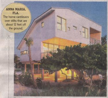
The home is made of poured concrete reinforced with steel rebar; its modernist design is intended to accentuate the fact that it is on stilts. Its height prompted its owners to decide against flood insurance.
